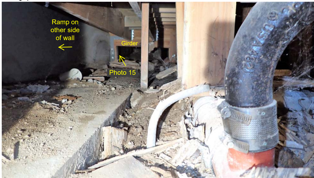
Photo 14: The crawlspace of the raised-floor viewing from the crawlspace opening toward the front. The floor joists run front-to-back, and the girders run left-to-right. The floor joists are attached to the girders with joist hangers. The ramp shown in Photo 5 is on the other side of the wall.
