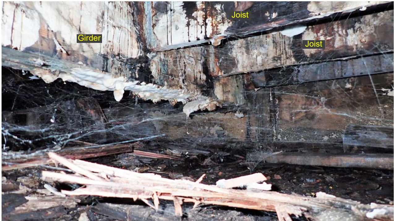
Photo 18: A closer view of the subfloor support framing below the cooler.
