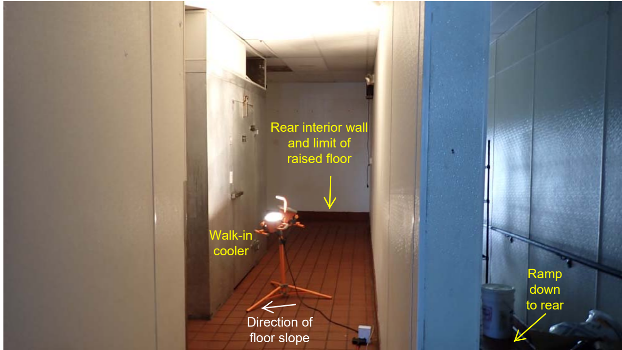
Photo 5: A view of the rear, raised-floor portion of the restaurant. The floor is covered with 6" x 6" square commercial tile. The cooler, which does not have its own insulated floor, is installed directly on the tile. The raised floor is sloping toward the cooler. There is a ramp toward the rear on the right side of the building.
