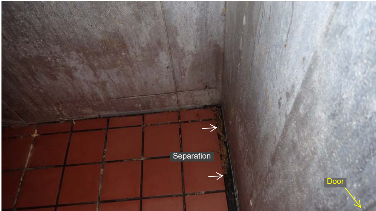
Photo 12: A separation between the tile and the front wall of the cooler.
