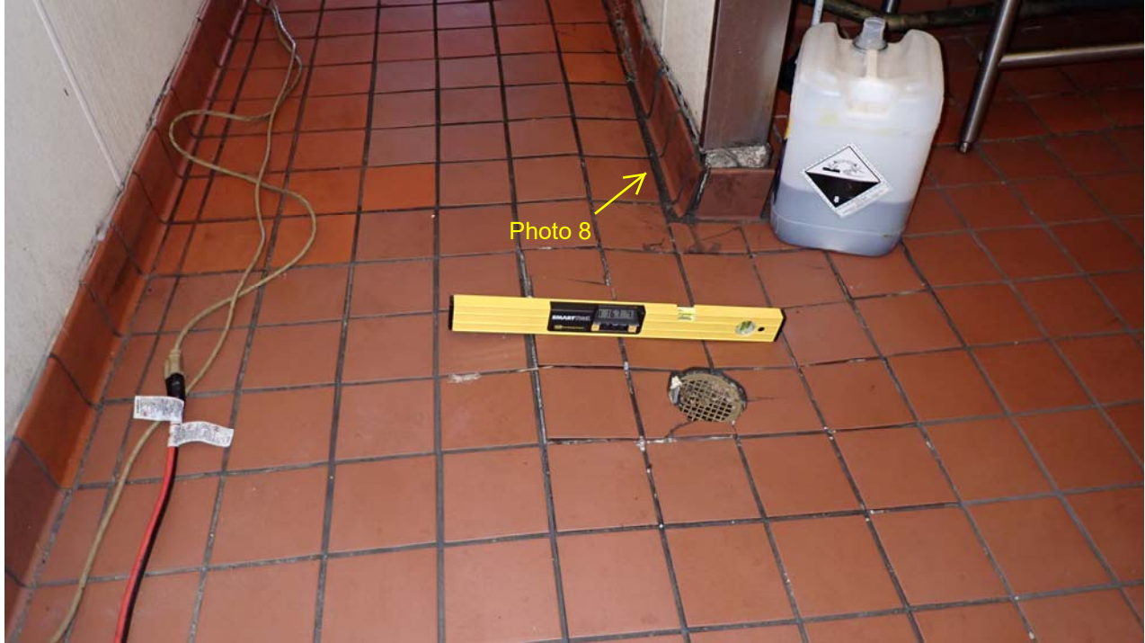
Photo 7: A closer view of the damaged raised floor. The floor feels weak and unsupported near the drain. The tile is cracked and loose surrounding the drain, and the cove base is separating from the end of the interior wall.
