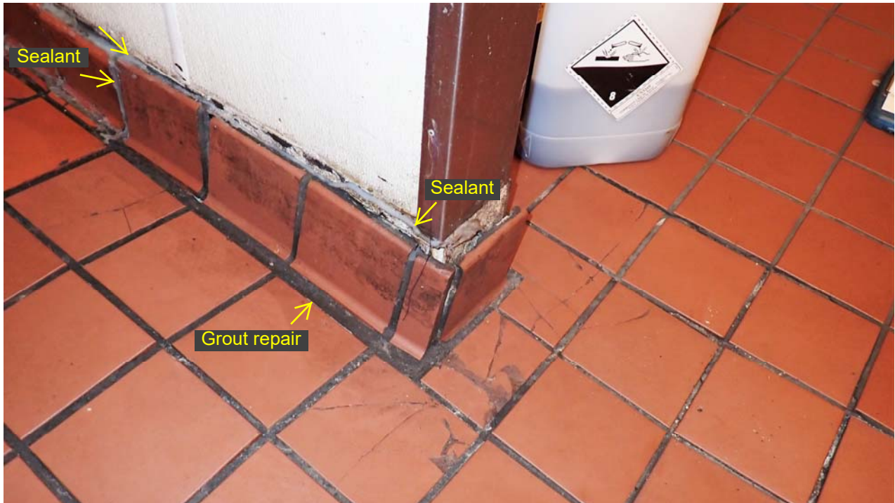
Photo 8: A closer view of the cove base tiles that are separating from the interior wall. Along the tiles, there is an older repair with sealant that has reopened.
