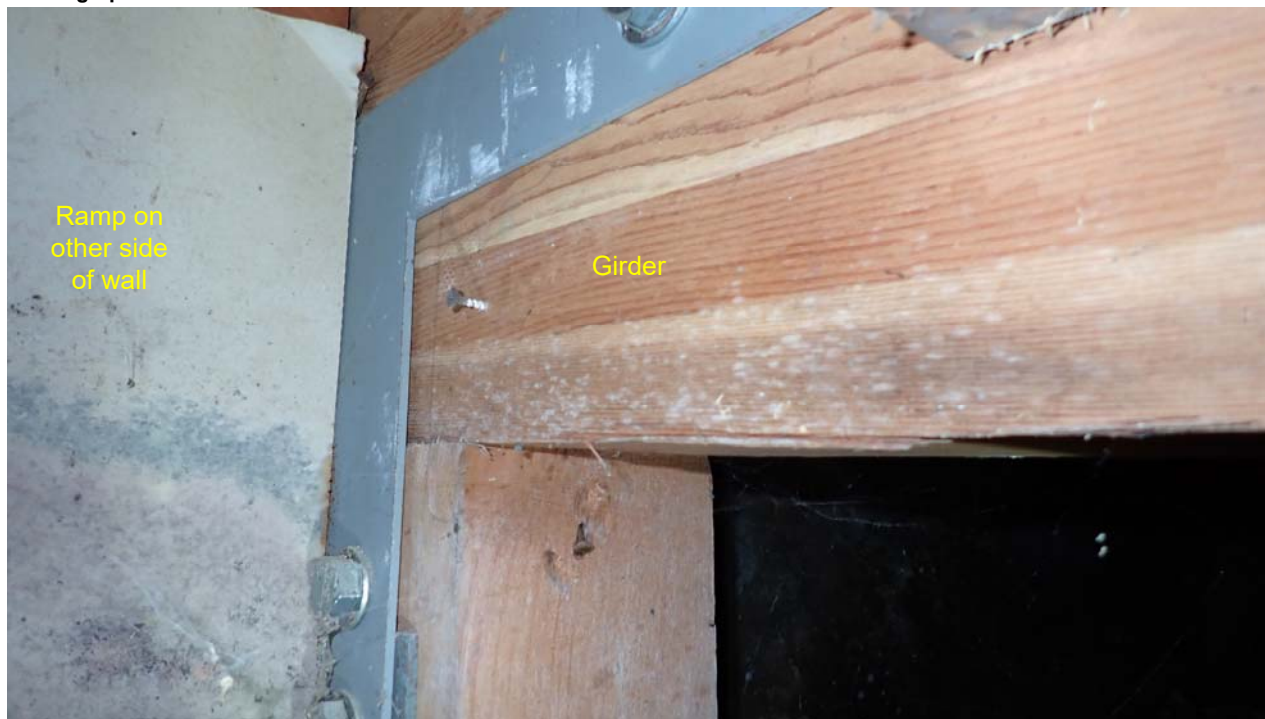
Photo 15: The girder shown in Photo 14 where it is supported on a post. The ramp shown in Photo 5 is on the other side of the wall. This framing generally appears newer than the construction of the addition in the mid 1960's, and there is construction debris throughout the crawlspace.
