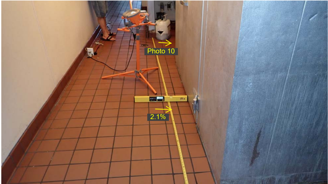
Photo 9: Another view of the tiled floor that is sloping toward the cooler at 2.1%.
