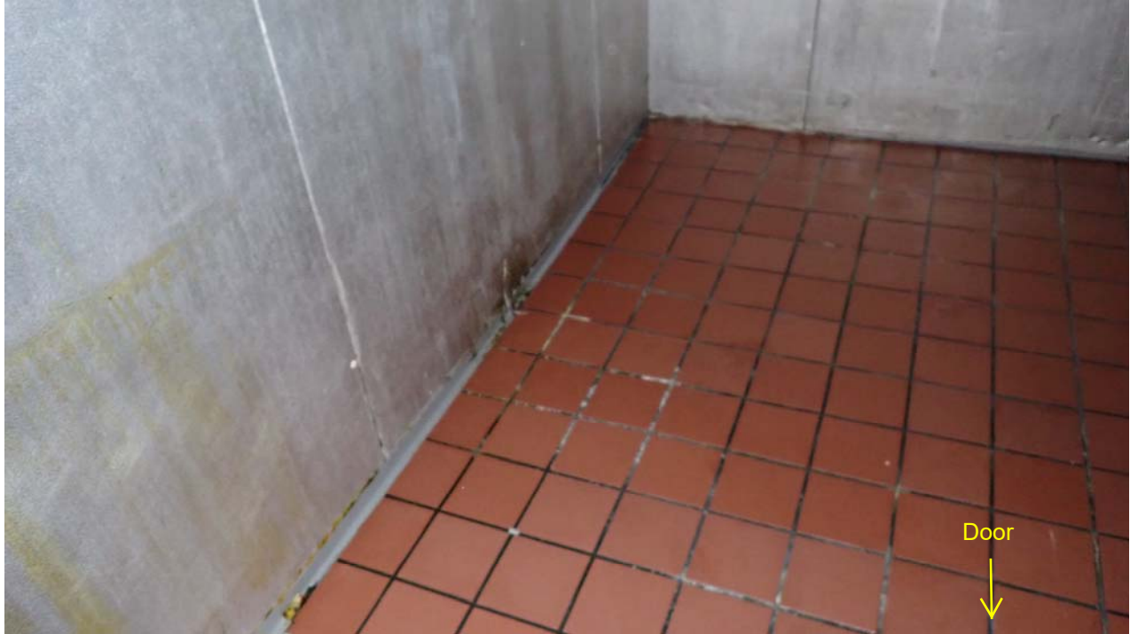
Photo 11: The inside of the cooler, which is installed directly on the tile without its own insulated floor.
