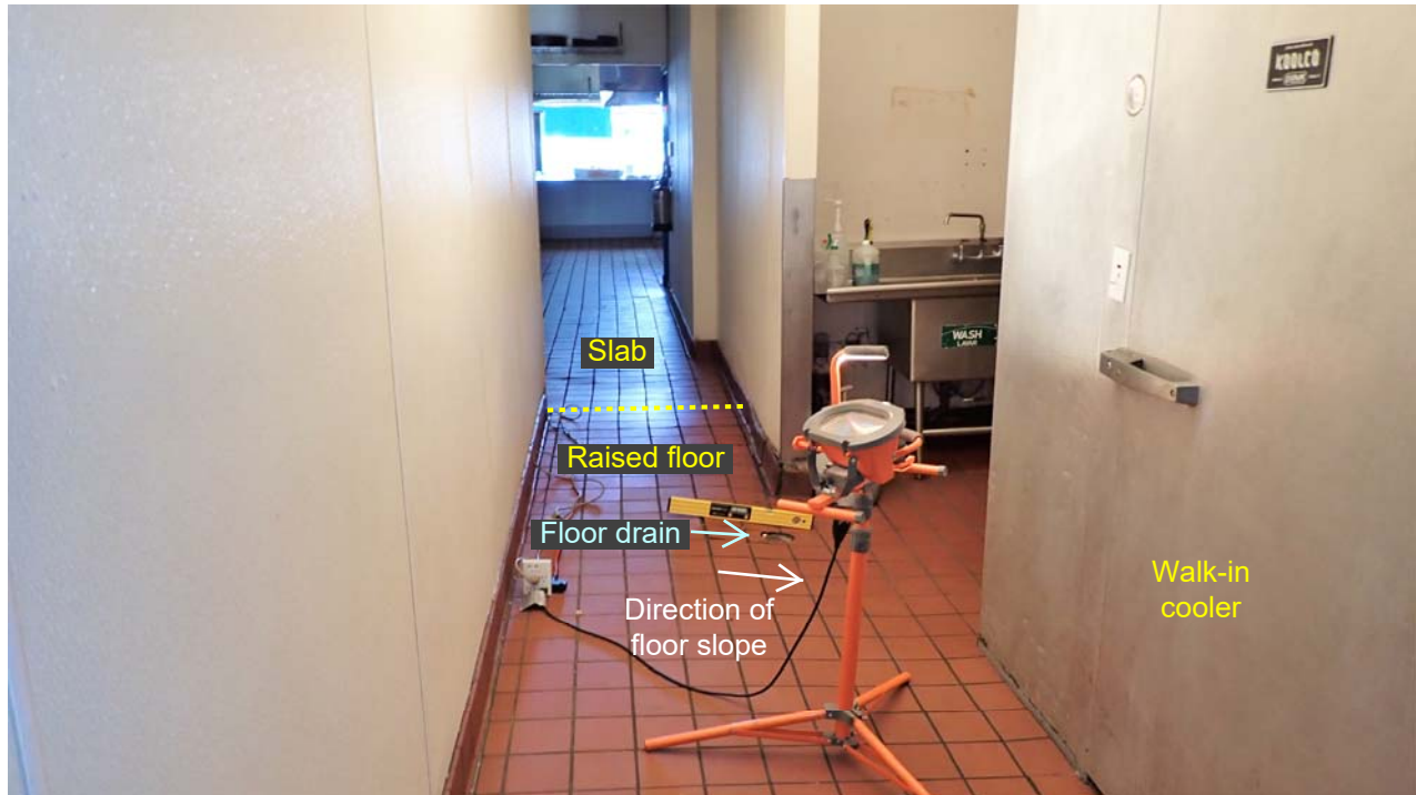
Photo 6: A view toward the front showing the walk-in cooler and the sloping floor. The slope of the floor increases near a floor drain.
