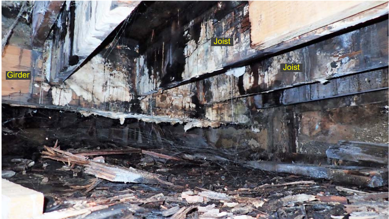
Photo 17: The framing below the cooler, which has severe white fungal blooms which have likely caused heavy deterioration and weakening of the floor support framing. The black substance, which has dripped over the white fungus, may be due to a past waterproofing attempt, or is some other unknown substance.
