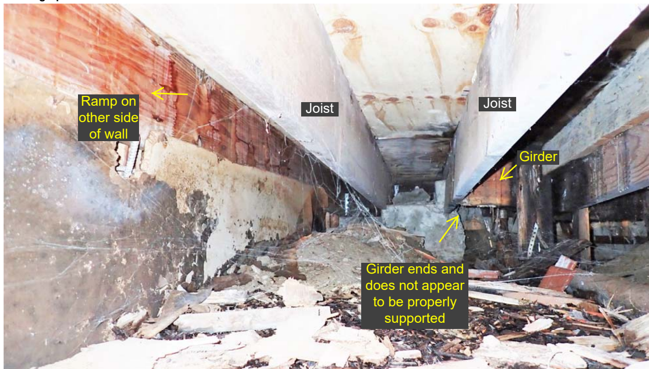
Photo 16: The crawlspace viewing toward the front just beyond the girder shown in Photos 14 and 15. There is abundant wood and tile construction debris in the crawlspace. Near the area shown in Photo 7, the girder stops and the end does not appear to be supported. Further exploration in the crawlspace was impeded by construction debris.
